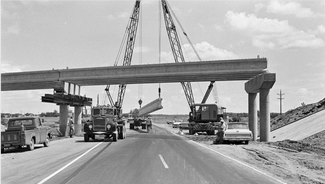
Interstate Highway 94, opened in 1968.
